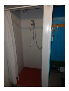
There is a shower cubicle in each changing room and also a toilet cubicle. The showers are operated by an electric shower unit. The shower water comes direct from the warm water heater housed in the plant room from a water pipe run at height through the ceiling above the changing room units.
